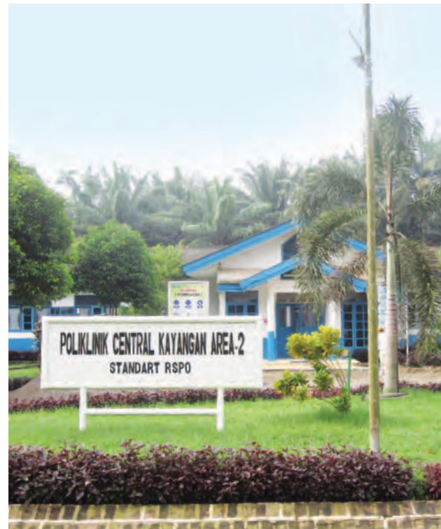
A clinic on site at Riau estate
