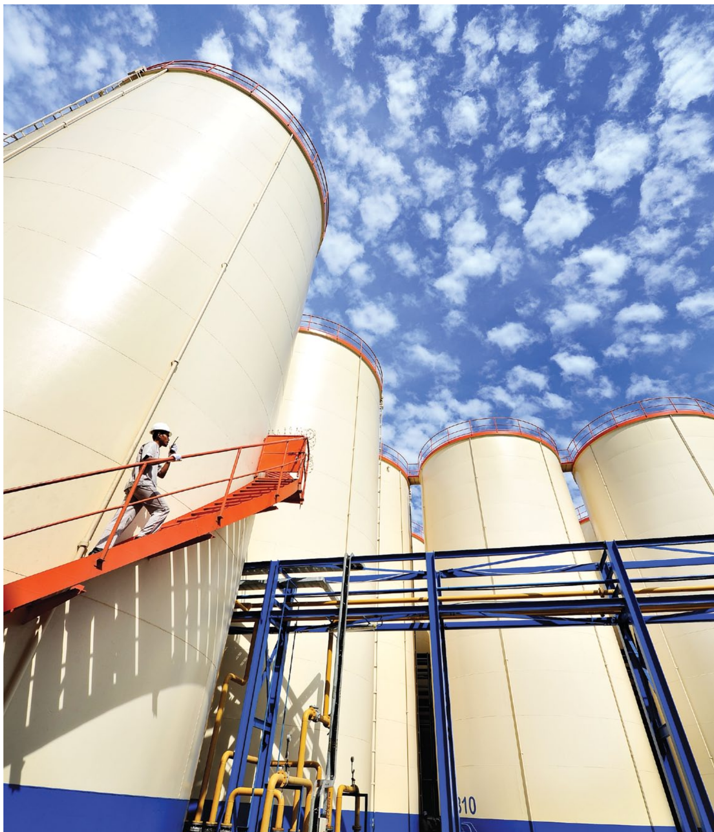
Storage tanks at Tanjung Priok Refinery
