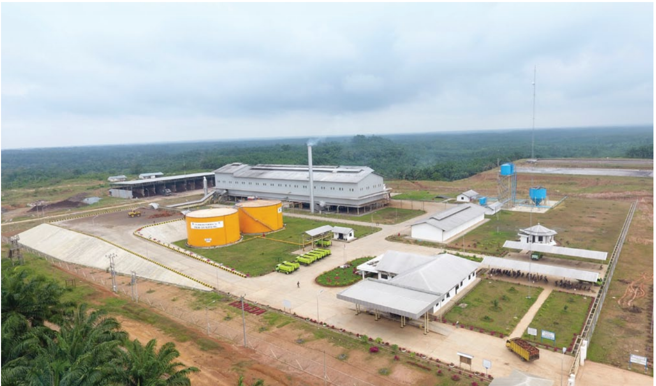
New Palm oil mill at South Sumatra
