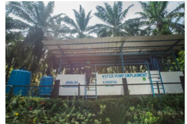
Water Pump Emplasmnt in Pulo Rambong Estate, North Sumatra
