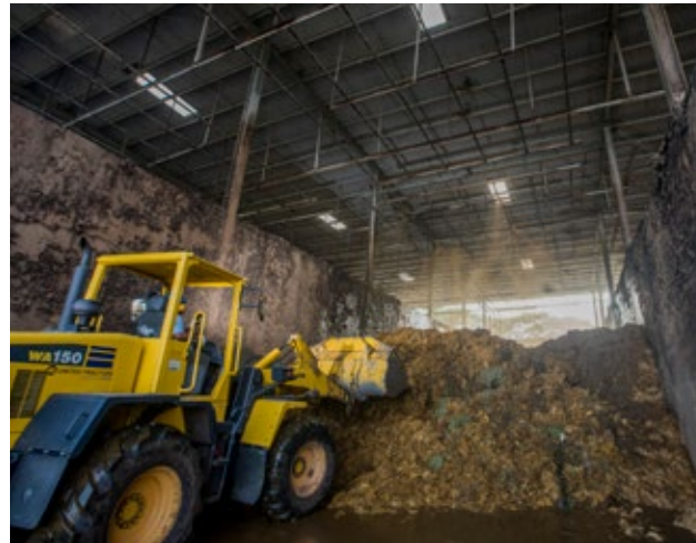
Aerated bunker composter at Dolok Mill, North Sumatra
